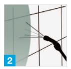
Wet the surface with the solution and leave for 10-15. Work in manageable areas at a time.
